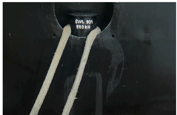
Sunken bitt with a sharp edge
