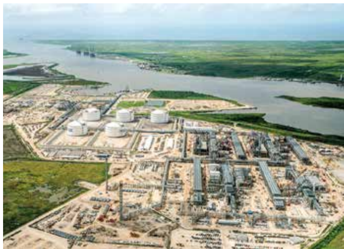
FIG. 1. Cheniere's Sabine Pass LNG complex is under construction.
