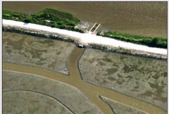
Over 300,000 smooth cordgrass planted in the tidal mitigation area
