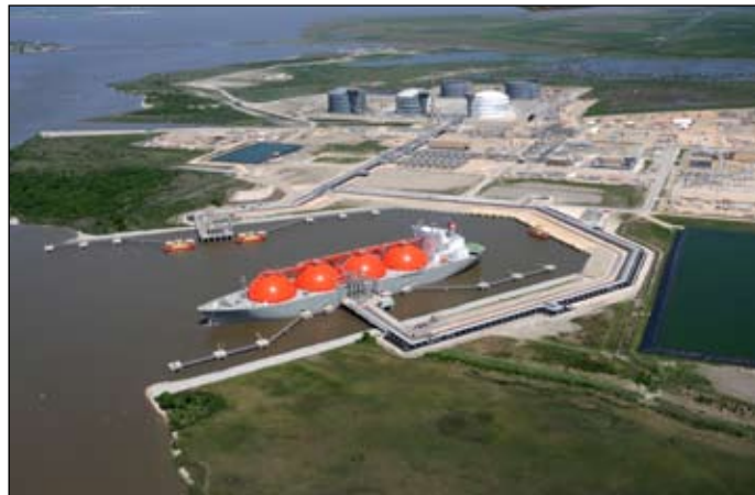
"Celestine River" sailed from Nigeria to bring the first cargo to the Sabine Pass LNG Terminal. (Moss sphere containment - 145,000 cm capacity)
